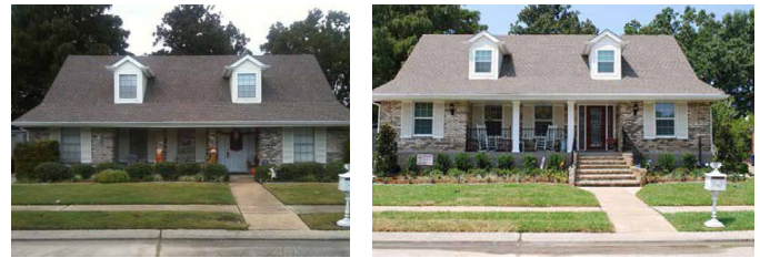
This ranch house was elevated to reduce flood risk after previously sitting close to the known flood risk level.
