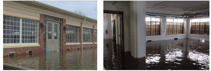
A building in Davenport, IA had vents installed at its base to allow flood waters to move in, through, and out of the building at a controlled rate.
